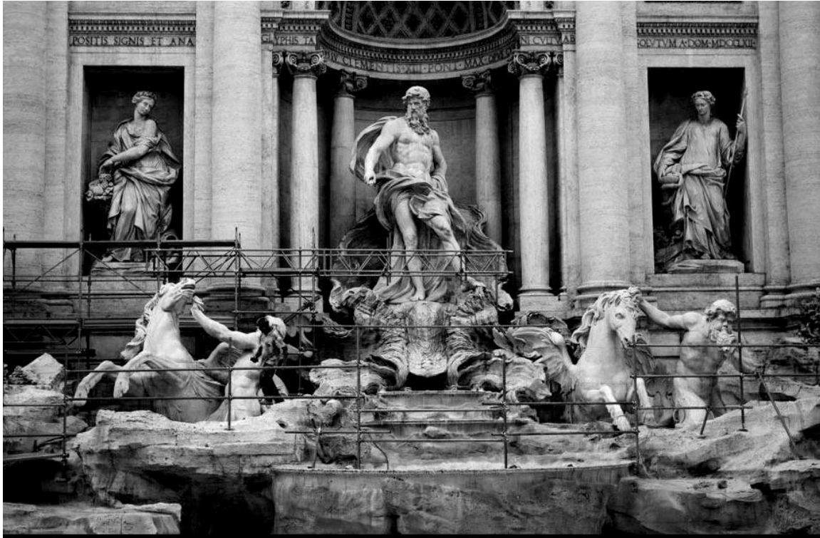
(figure 3: restauration works in Fontana di Trevi, 2013)
